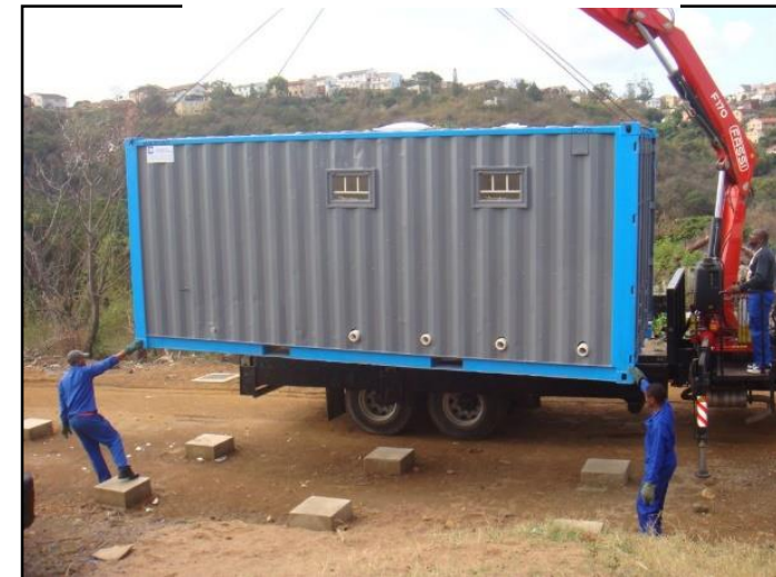
Communal Ablution Block
